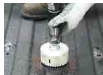
Use the pilot hole for error-free drilling
